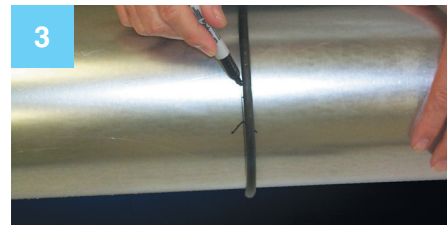
Use O-ring provided and mark for cut.
