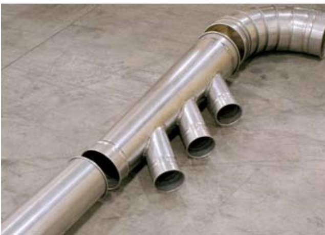
Lay your system out on the floor
