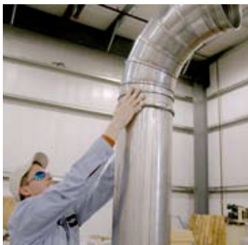
Lift pieces into place
