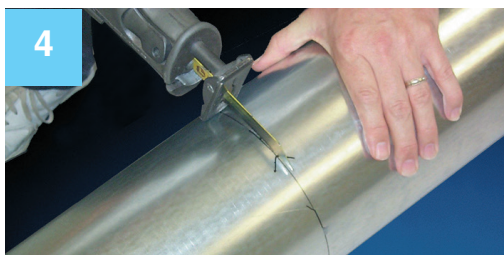
Drill access hole, then cut the QF Pipe.
