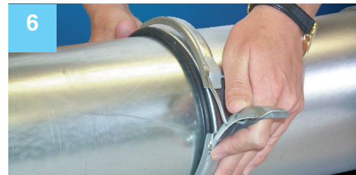
Snap QF Clamp over the QF O-ring and end of QF Adjustable Nipple.
