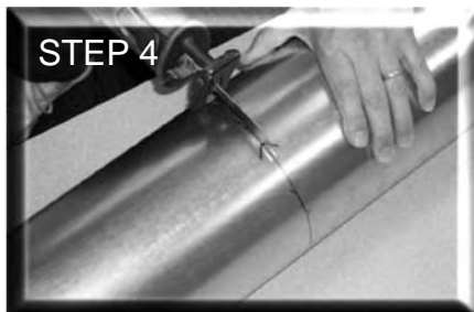
Drill access hole then cut with saw
