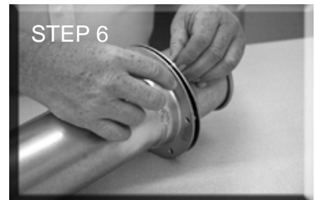
Connect the two flanges with the provided nuts and bolts
