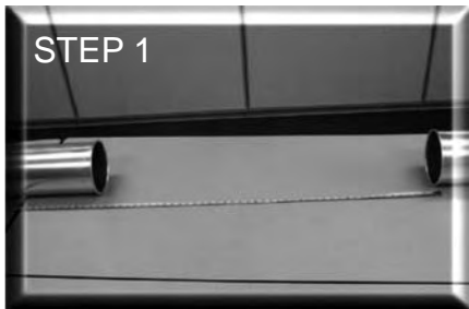
Measure distance to be spanned.
