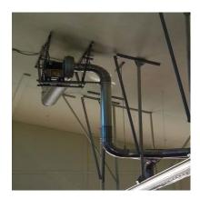
The most effective method of limiting the exposure to diesel exhaust is the Exhaust Source Capture System. Inside the fire station a pneumatic nozzle, connected via hose to a ducting system above, is attached to the Fire truck's tailpipe where it captures the fumes and then easily pulls them out of the building.
